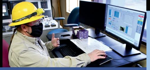
**Above** John Naber, electrical and control, Corn Belt Power Cooperative, displays the new interface on one of the new HMI computers at Wisdom Station. The computers help to access and troubleshoot the Wisdom Unit 2 control system.
